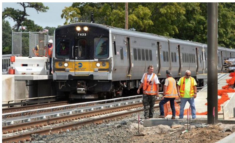
Second track construction between Farmingdale and Ronkonkoma. Image source: Newsday.
