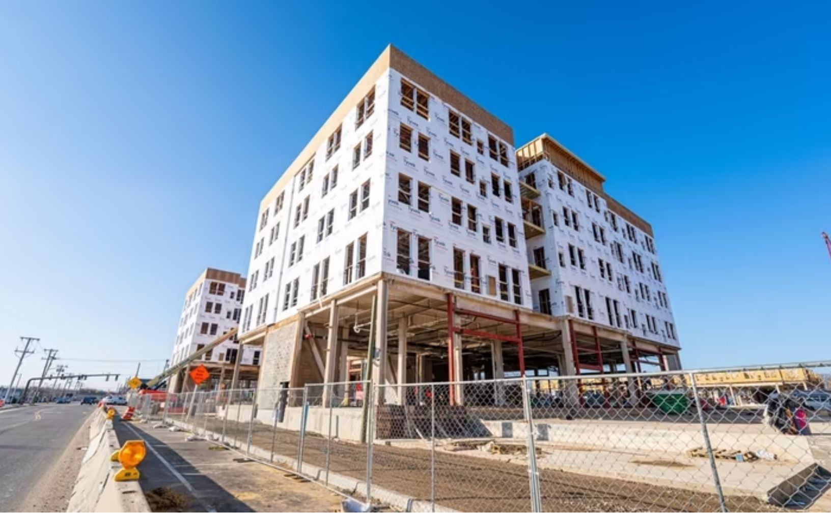
Station Yards in Ronkonkoma. Image source: Newsday
