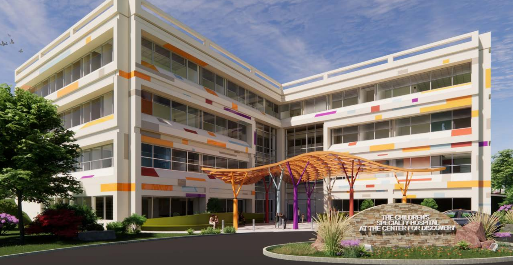
The Center for Discovery, Children's Specialty Hospital Rendering, Rock Hill, Sullivan County
