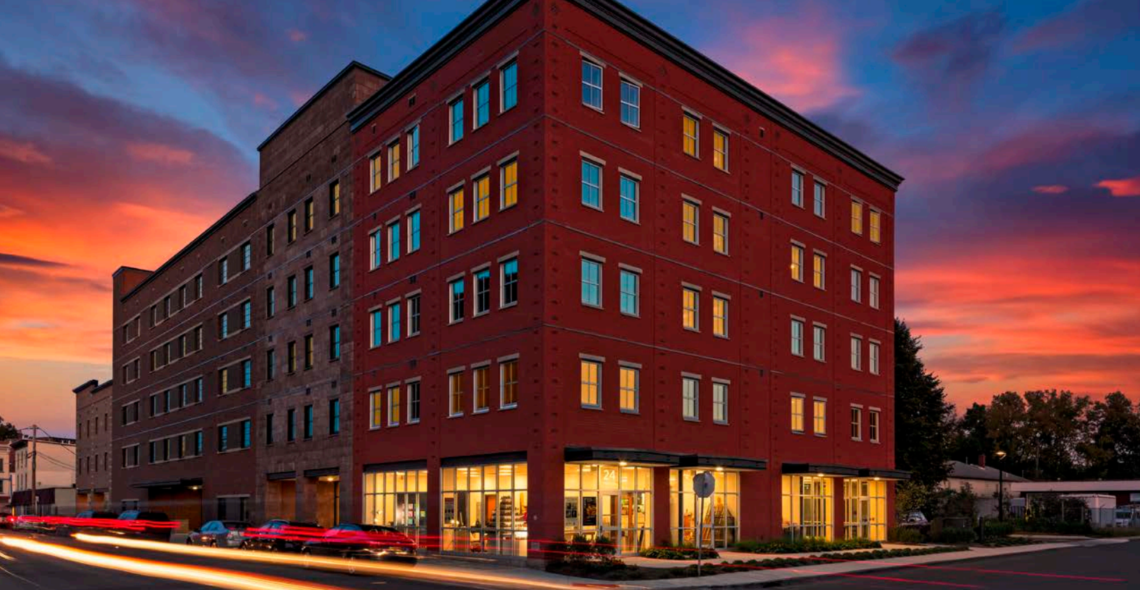
Energy Square, City of Kingston, Ulster County
