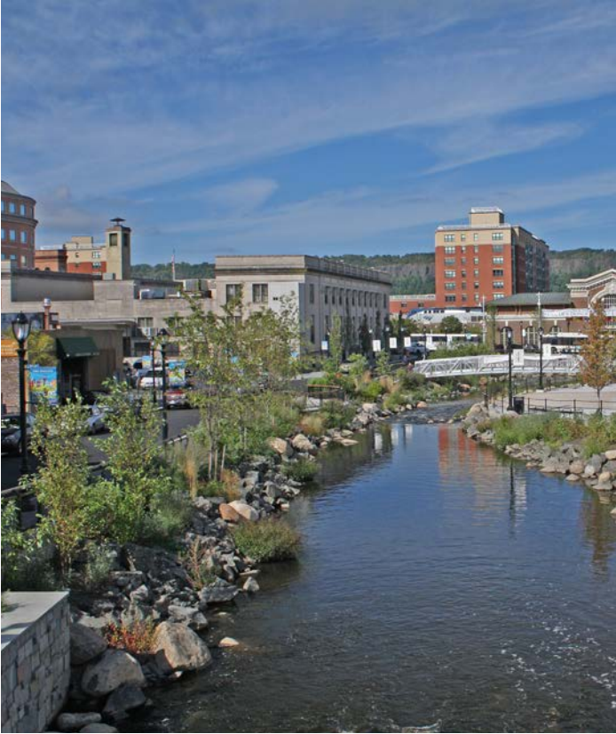
Saw Mill River Daylighting, Yonkers, Westchester County
