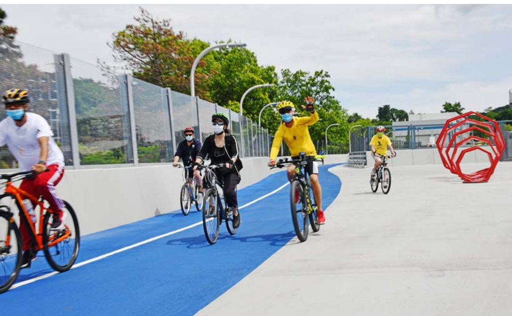
Shared Pedestrian Walkway, Governor Mario M. Cuomo Bridge
