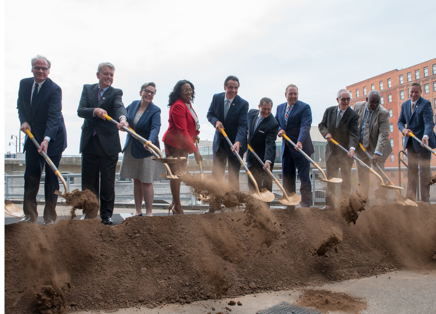
Officials break ground for ROC the Riverway at the Convention Center north terrace improvement project.
