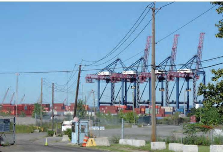
Howland Hook Marine Terminal entry gate and container cranes
